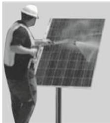
Use a hose with a suitable nozzle to allow the stream of water to reach the panels.
