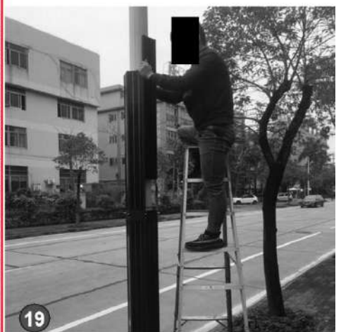
18 Connect the MC4 connectors and put it back inside of the module tube. (It will be invisible from outside.)
