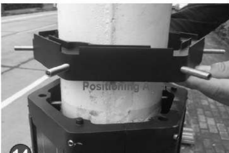
13 Fasten the 6 pieces screws with driver carefully.
