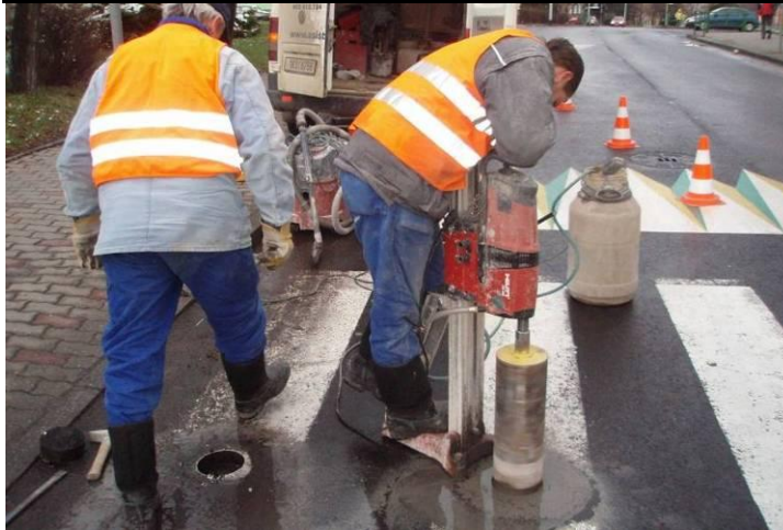
LightMark S2X – Crosswalk Installation
