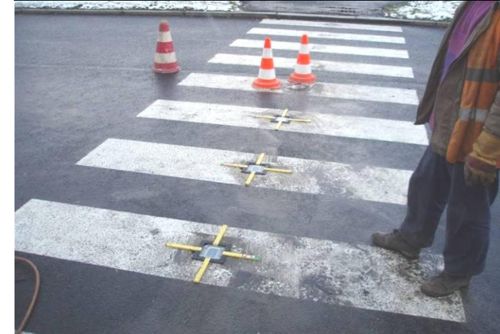
LightMark S2X – Crosswalk Installation
