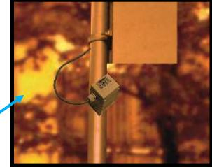
**Step 5 B** For the radar cable, you need to first attach the radar to the pole, orienting the sensor to the crosswalk as seen in the picture.
